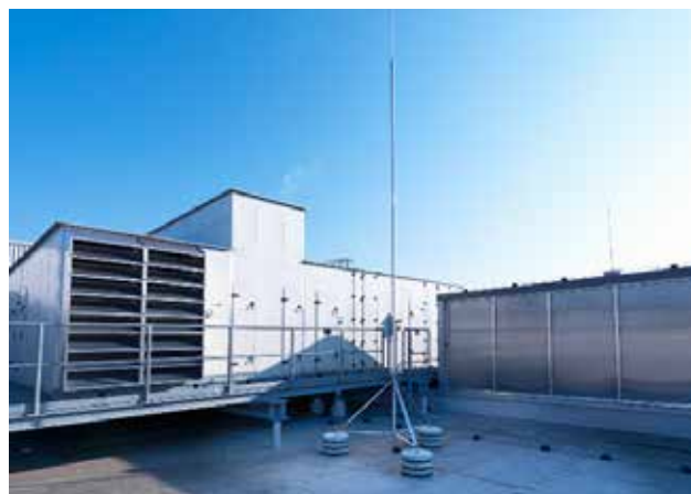
Fig. 2.29: Aluminium air-termination rod
