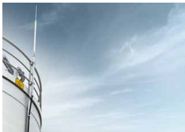
Figure 2.58: Isolated lightning protection with isCon®
