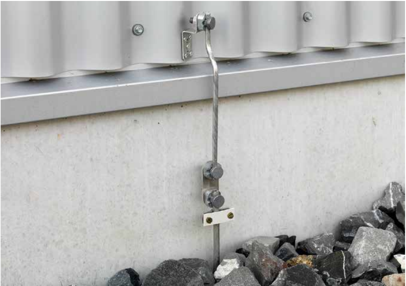
Figure 4.1: Separation point on a metal facade
