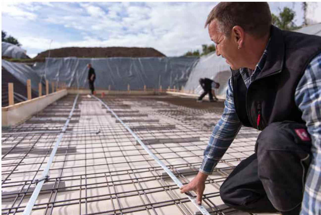
Figure 2.75: Installing a foundation earther
