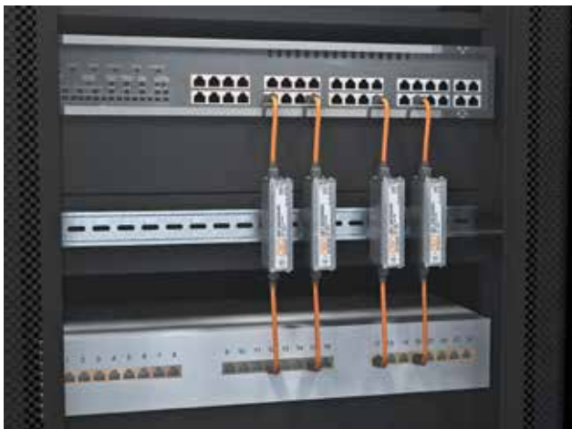
Figure 3.81: Suggested protection for switch with patch panel. The surge protection devices are earthed via the hat rail.
