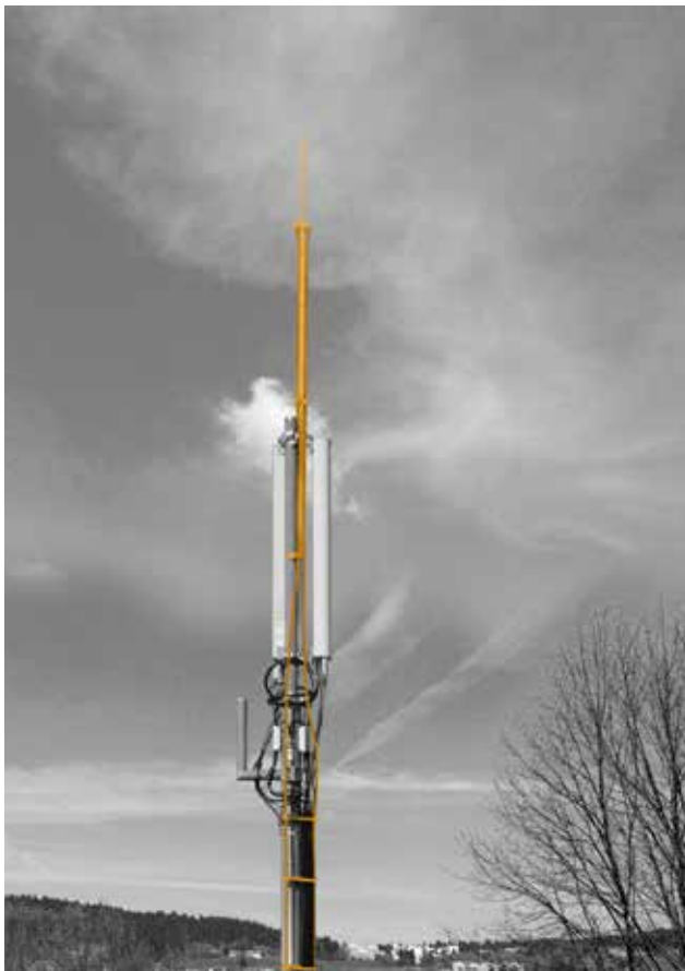
Figure 2.72: Cell tower with isCon® conductor
