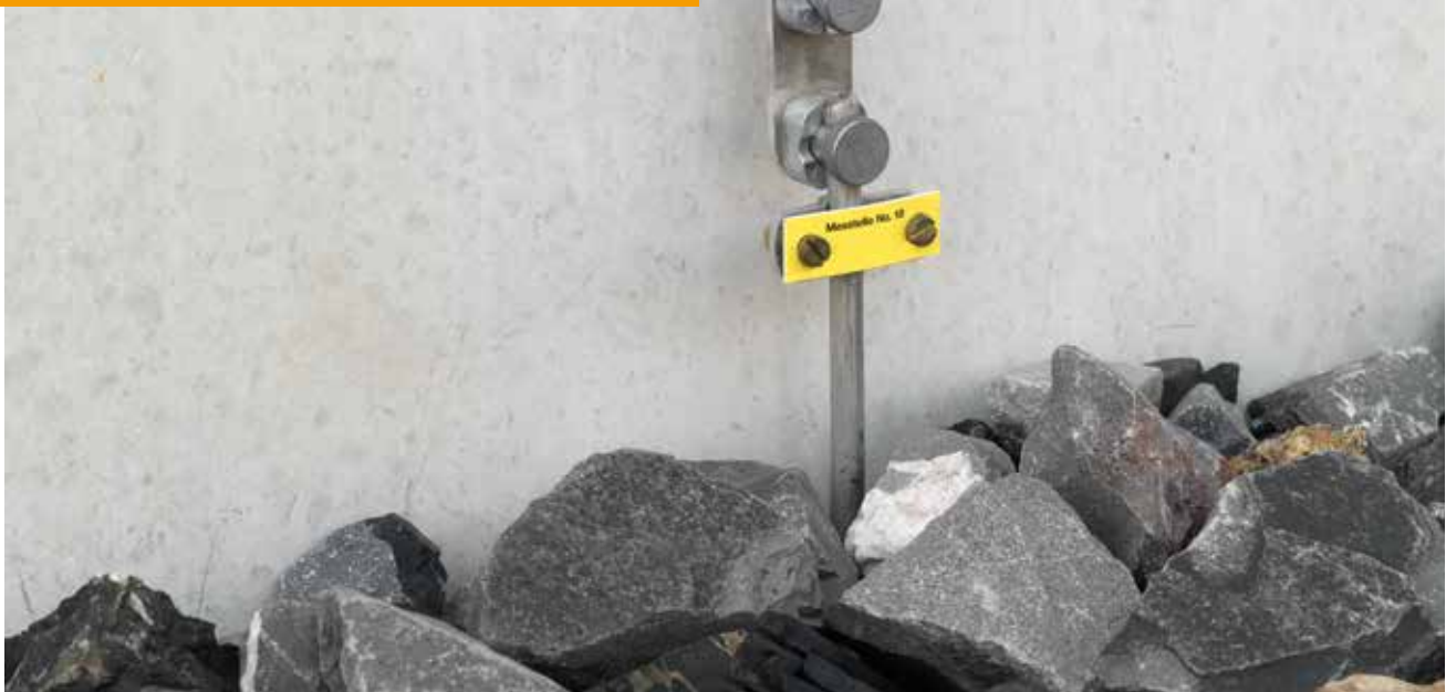
Figure 2.48: Measuring point at the point of entry into the earth
