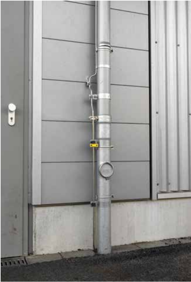
Figure 2.18: Lightning down-conductor at a downpipe
