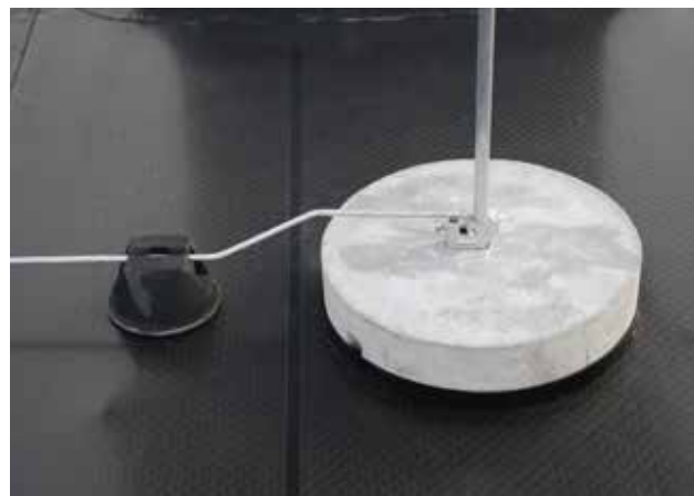
Figure 2.22: Air-termination rod
